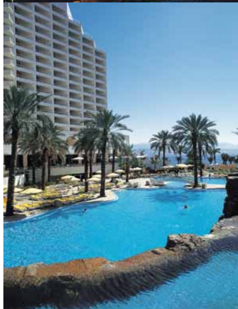
Princess Eilat Hotel. Under reconstruction currently.
